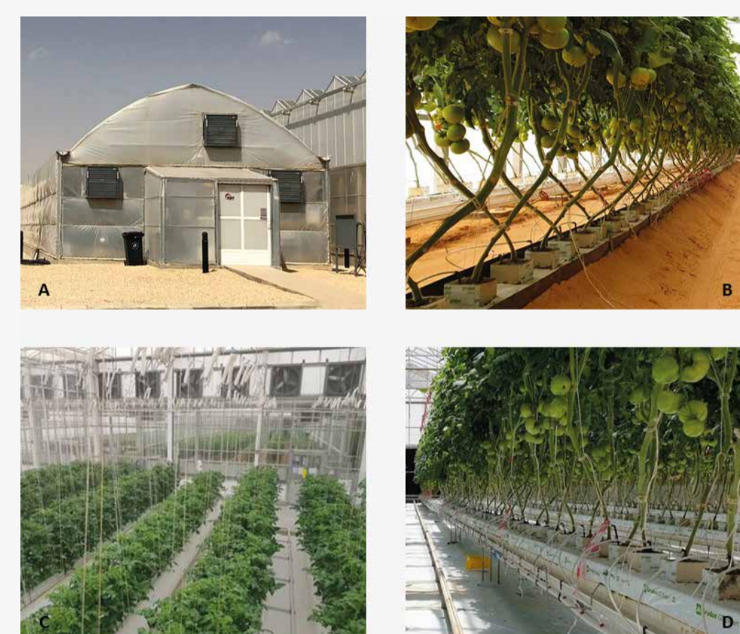
Figure 1. View of the greenhouses. The L plastic tunnel from outside (A) and inside (B) and M glass Venlo greenhouse (C and D) where the exhaust fans are placed higher (C).
